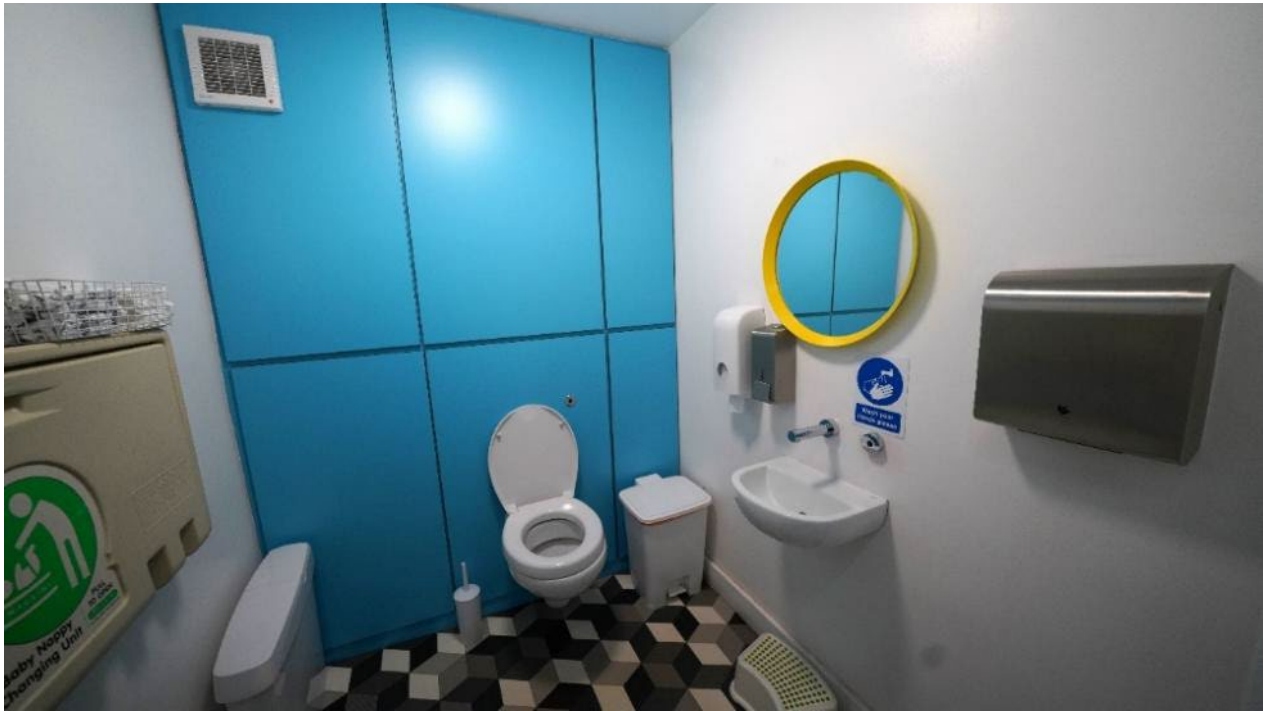
Floor 4: Unisex toilet interior
